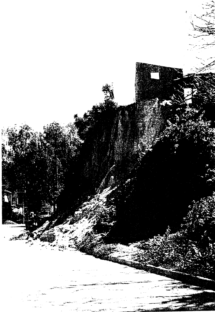
Figure 11 Fall in near-vertical cutting causing collapse of house, Santiago Texacuangos.
